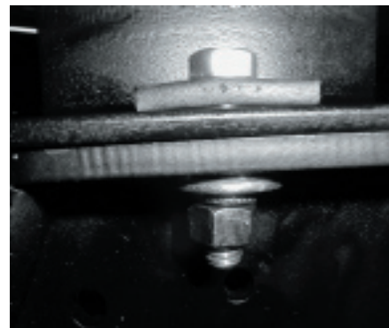
GRADE 5 BOLTS USE ONE 1" X 2" PLATE WASHER AND TWO 1/2" FLATWASHERS
