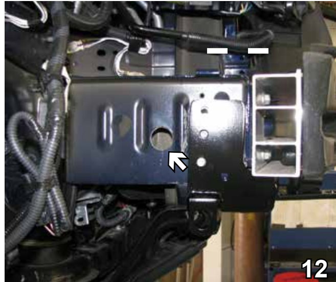
12. Drill a 1 1/4" hole in the area shown which will be used to insert nut plates. Do this on both sides of the vehicle.
