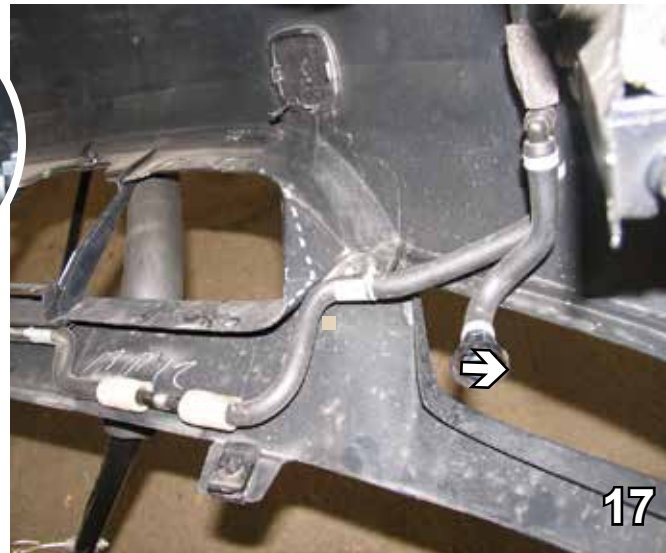
17. Before reinstalling the bumper, connect the head light washer hose. Reconnect the fog lights and running lights.
