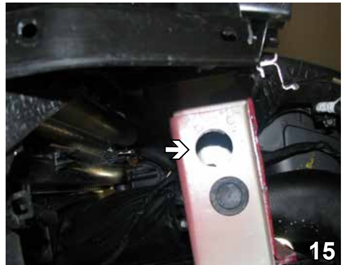
15. Underneath the frame, using a 1 1/4" hole saw, drill a hole in the bottom of the frame for the nut plates. Do this to both sides of the vehicle.
