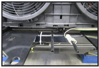
13. Install the wire loom cover around the condensor lines to prevent rubbing (left). And zip-tie the line to the baseplate to prevent it from moving around (right).
